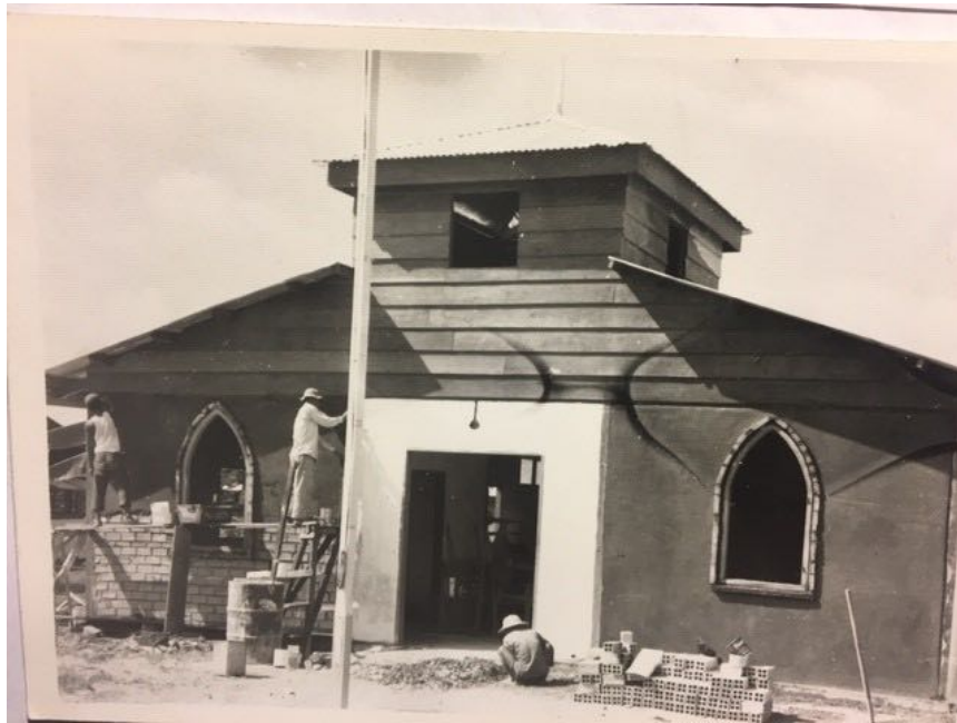
Chapel construction nearly complete
